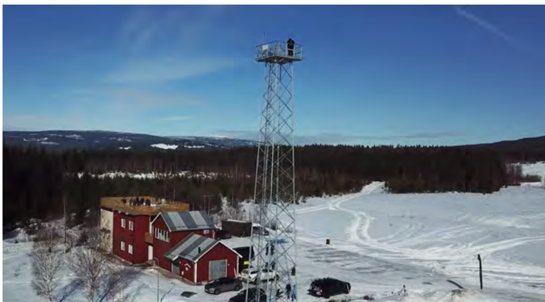
Figure 2.2 An overview of the main command buildings at the ICE worx Rena site.
